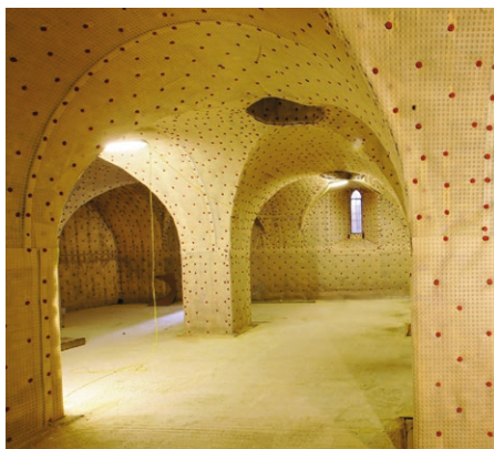
Figure 1: Newton cavity drain membranes were effectively applied to the interior vaults of the Grade 1 Listed Royal Courts of Justice, London. Here we can see the completed system, prior to the application of the internal finish.
