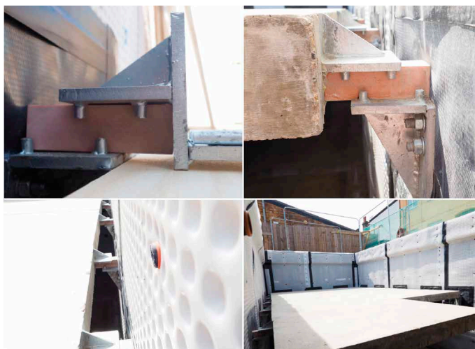
The bespoke brackets, designed by Joe and his structural engineer, allowed for the installation of the ingenious ‘floating’ slab
